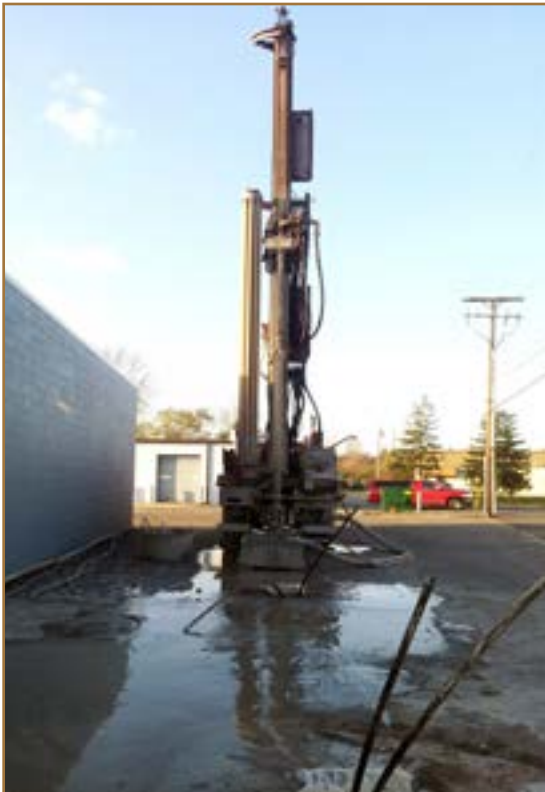
Figure 1, Geothermal Drilling
