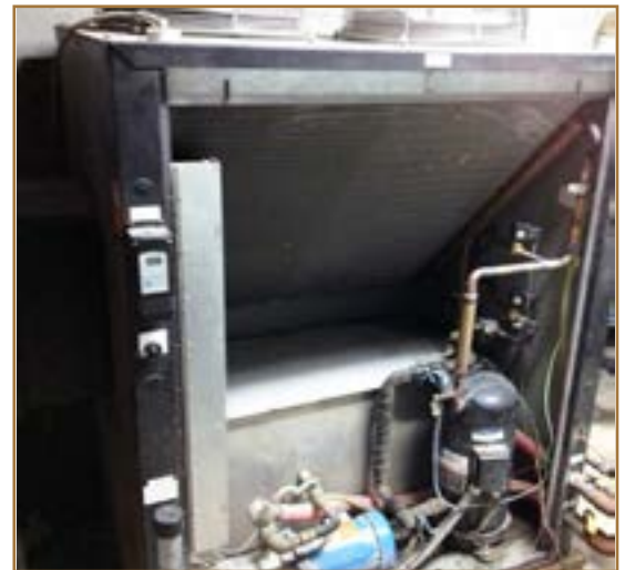
Figure 3, Refrigerated Water Cooler
