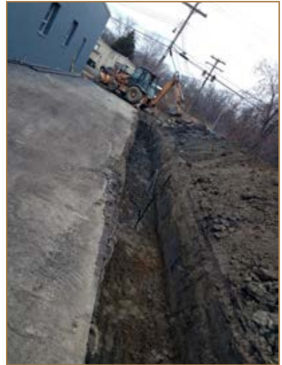
Figure 5, Empty Pipe Trench
